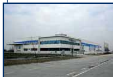
PSM Facility Grand Opening 2010
